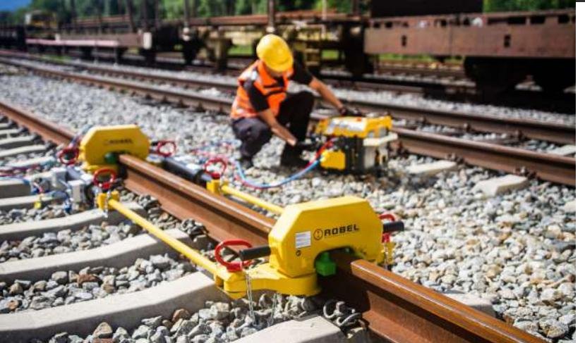
**The modular concept for creating a neutral rail tension during welding and bracing work.**
