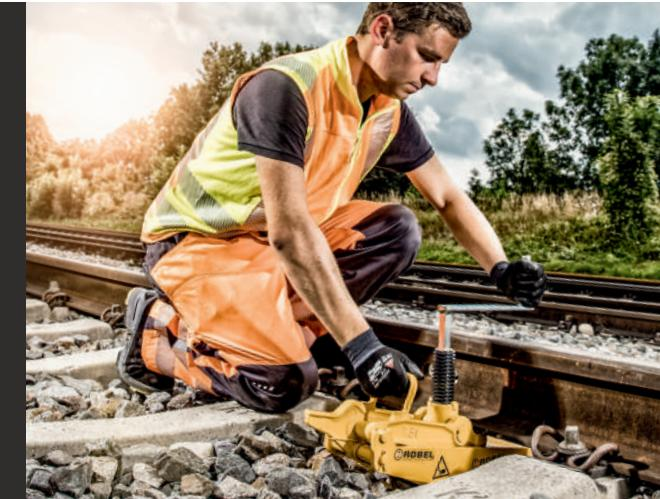
**For precise lifting of rail.**
